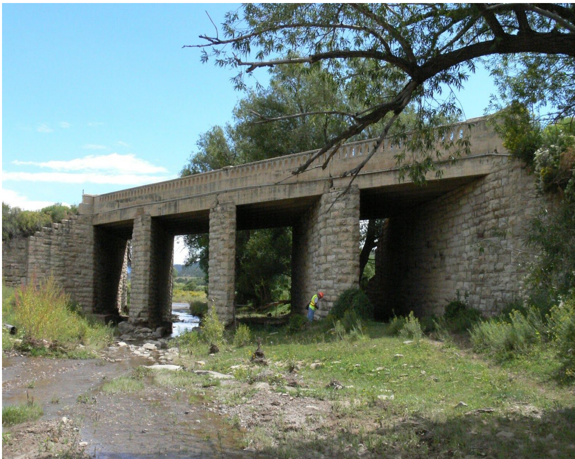
Zaracillo Canyon Bridge
