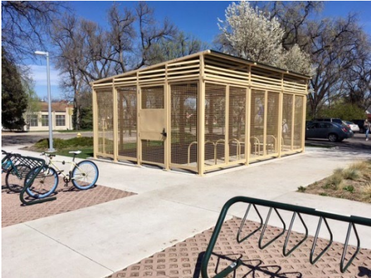
Above: Secure bike shelter at University Ave MAX Bus Station on CSU Main Campus in Fort Collins. Paid registration is required for access. Credit: CSU
