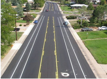
Above: Attached (no buffer), Rollover Curb
