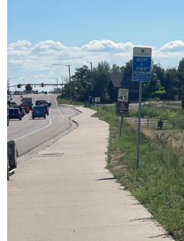
Above: Attached (no buffer), Vertical Curb
