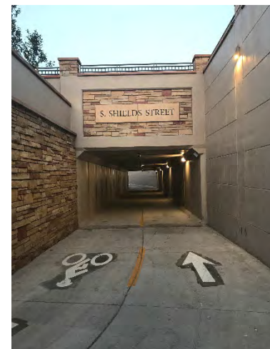
Above: Underpass at Shields Street in Fort Collins
