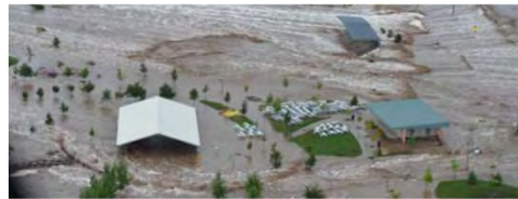
Water cascading over the railroad and Railroad Avenue and into Fairgrounds Park during 2013 flood. The railroad acts like a dam, ponding water upstream due to conveyance limitations and eventually overtopping and flooding property downstream.
