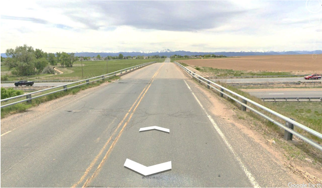
WCR 38 at I-25 Street, view west
