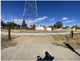
Tennessee Ave Shared Use Path: Gap between curb cut and shared use path
