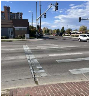
Federal & Louisiana: Large intersection with no medians or other shelter for crossing pedestrians
