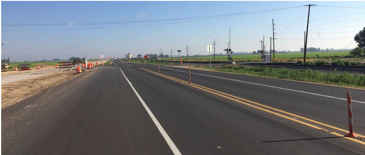
Image 3-2: Construction at US85 and SH392 (CDOT)
