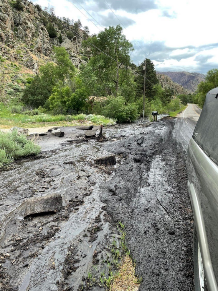
Image 2-6: Post-fire debris flow running onto SH 14. Image credit Coalition for the Poudre River Watershed.
