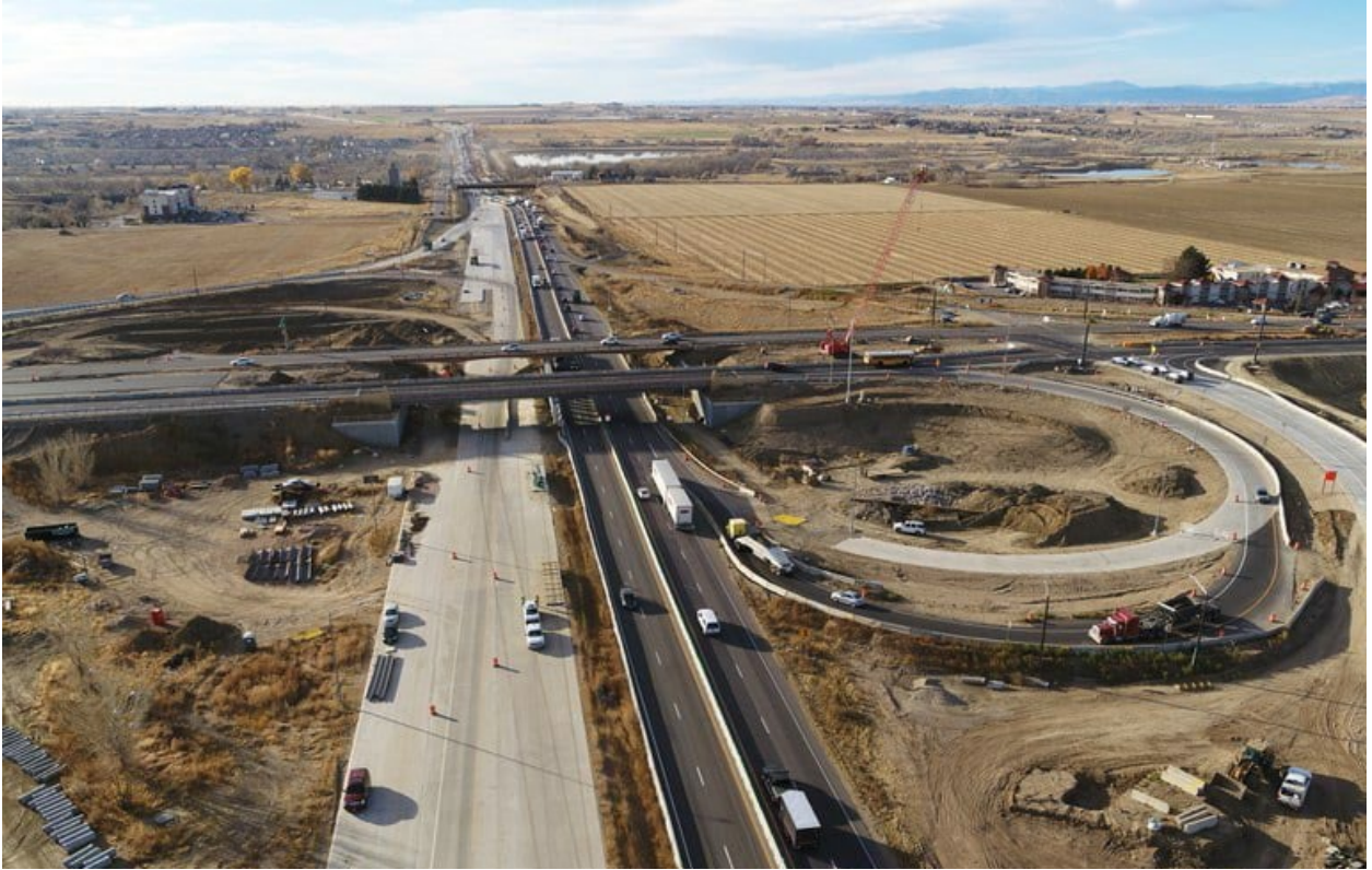
Image 3-1: Construction at I-25 and US34 in Loveland (CDOT)
