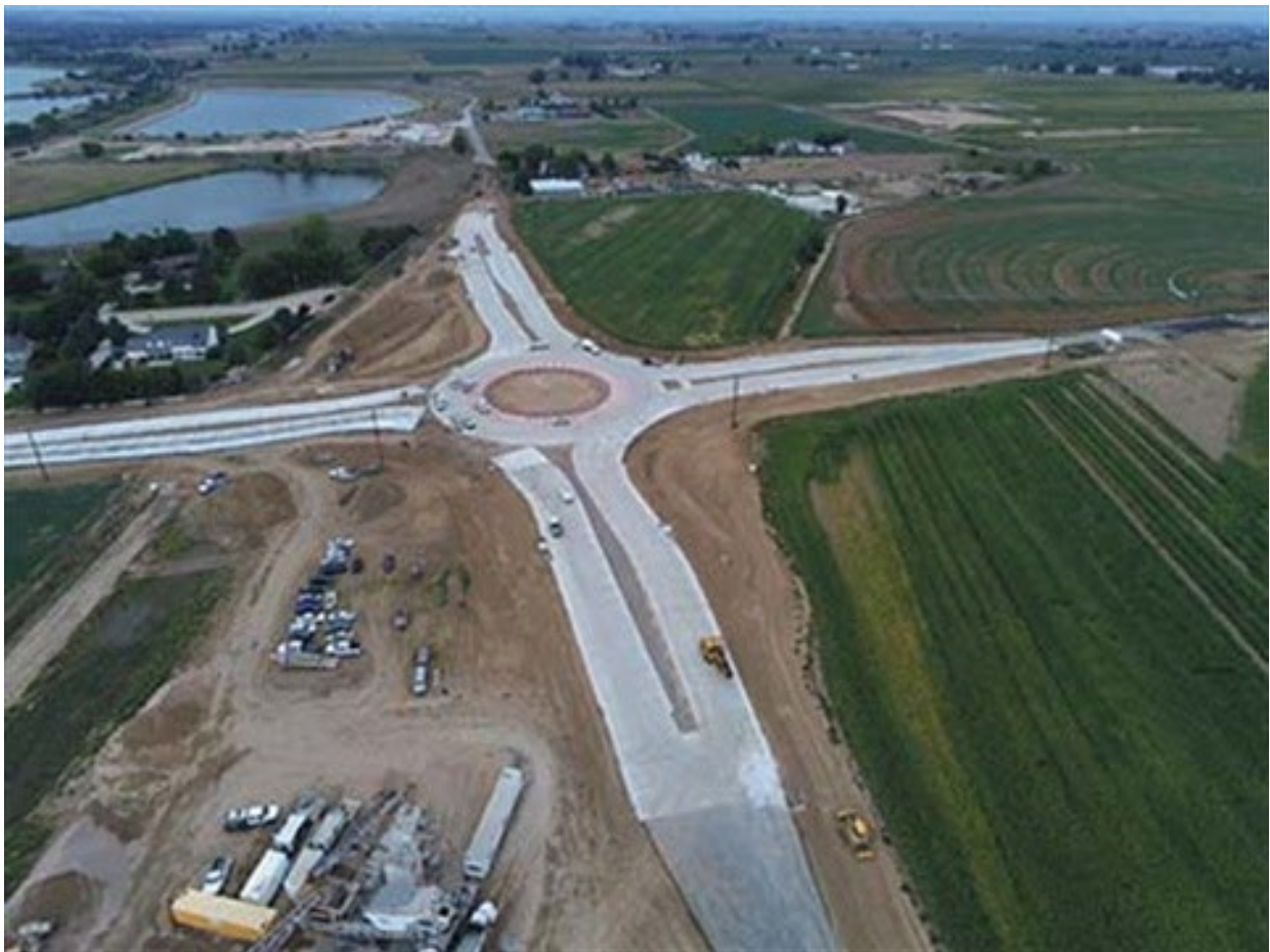
Image 3-11: 35th Avenue and O Street roundabout construction (Weld County)
