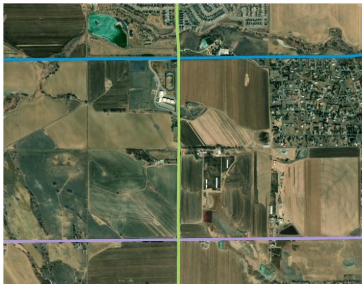
Figure 3-32: Location of the road widening project between 37 th Street (blue) and 49 th Street (purple) in Evans/Weld County set to begin construction in 2027
