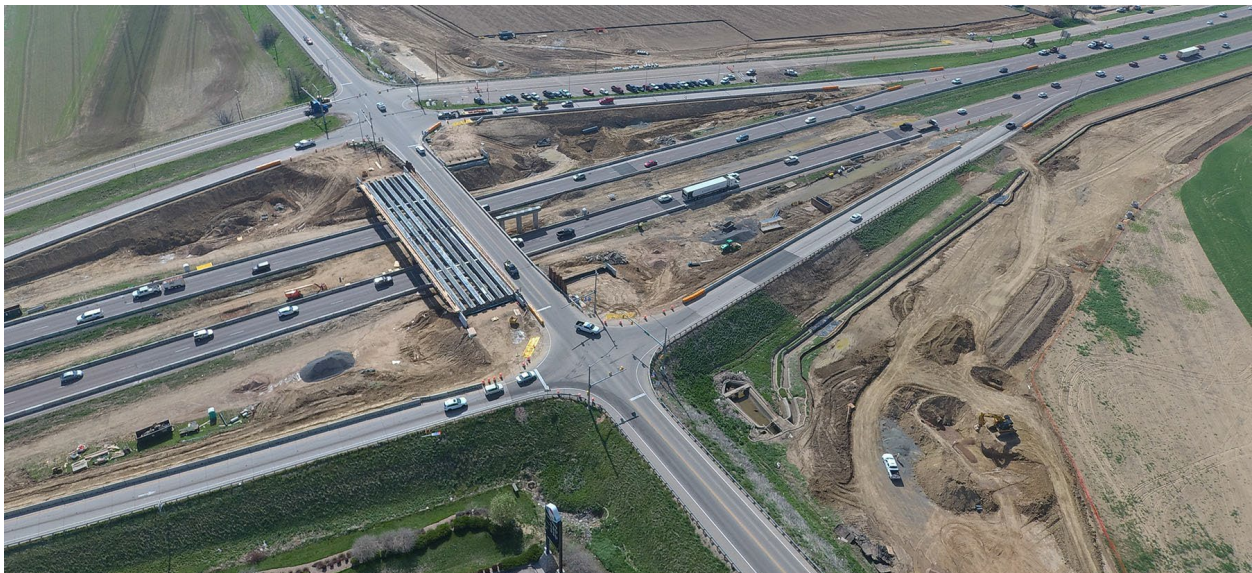
Image 3-7: Construction at SH60 and I-25 – May 2021 (CDOT)
